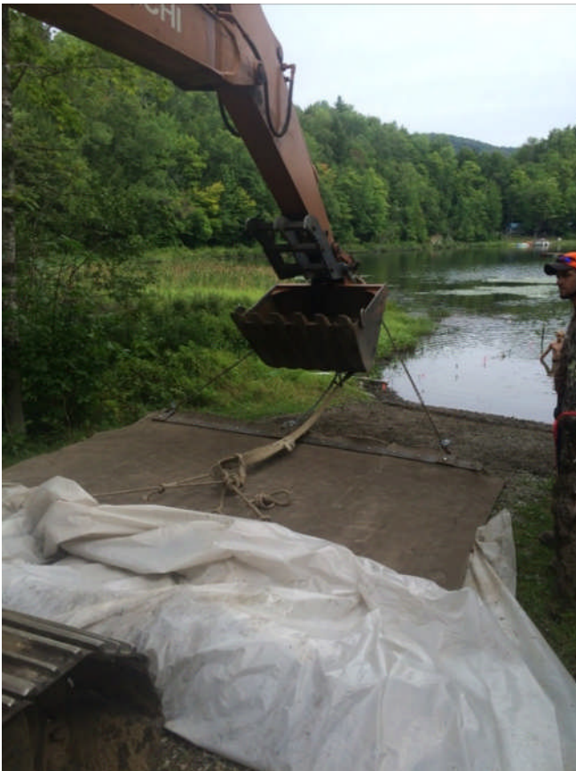
Figure 4. Concrete cloth being dragged into place on the gravel bottom of the Dog Pond Access Area, Woodbury, VT, August 2016.
