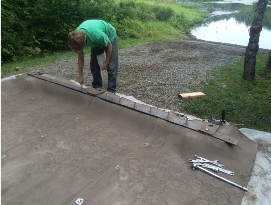
Figure 3. Bolting the 4 ft. strips of concrete cloth together prior to setting it in place at the Dog Pond Access Area in Woodbury, VT.
