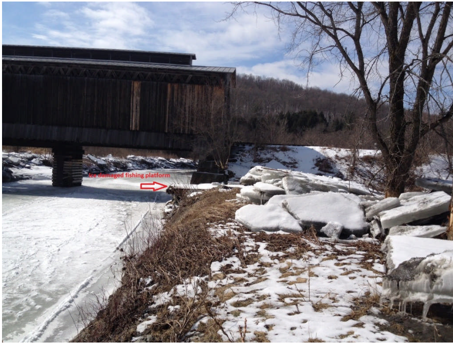
Figure 1. The 10x20 Fisher Bridge fishing platform on the Lamoille River in Wolcott was damaged following heavy February rains and subsequent flooding. Sheets of ice greater than 20 ft. across floated down the river, shearing off the platform's railing. The railing was replaced in June 2016.
